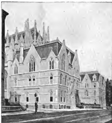
ARCHBISHOP'S RESIDENCE, ST. PATRICK'S CATHEDRAL, MADISON AVENUE AND 50TH STREET.
